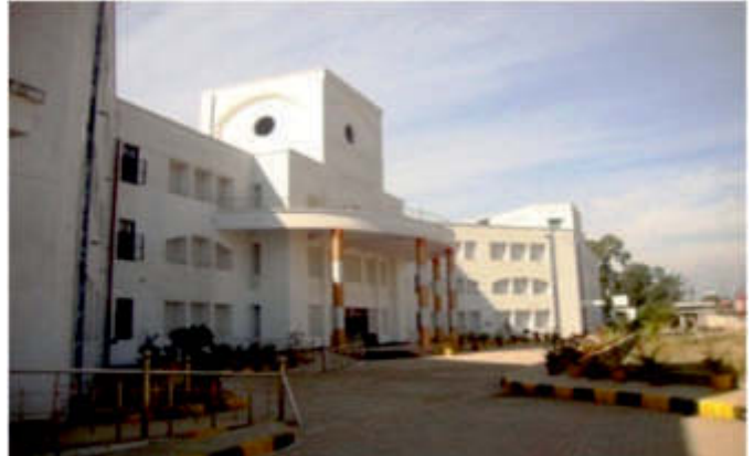
Newly Constructed Building of KV IIP, Mohkampur, Dehradun (Uttarakhand)
